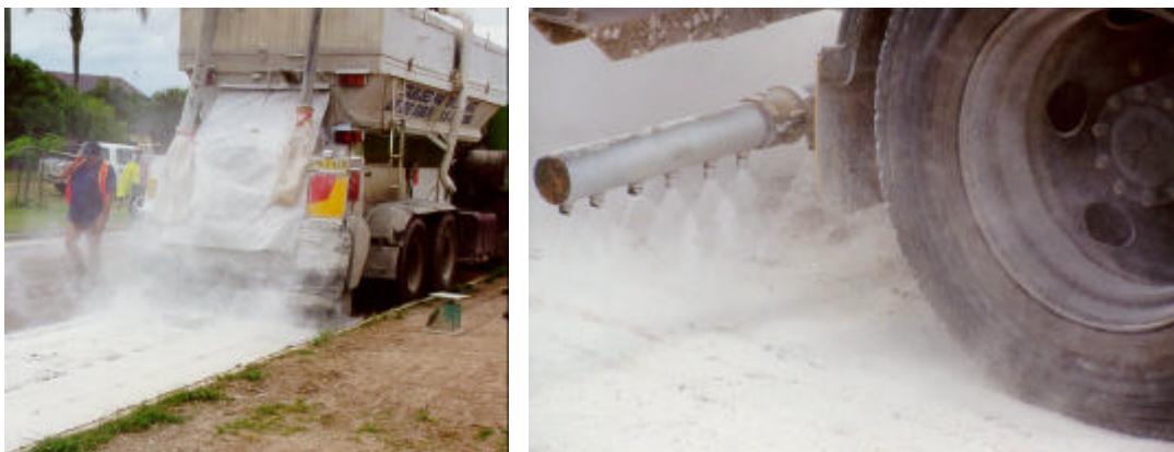
Figure 3 – Spreading (left) and slaking (right) of quicklime
