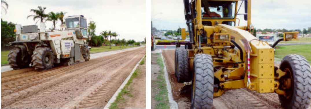
Figure 2 – Pre-milling existing pavement (left) and shape correction (right)
